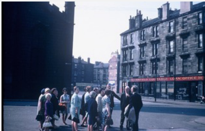
Figure 1: Annie's Loo, One of the First Tenement Retrofits
